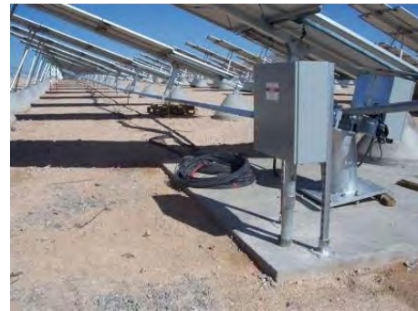
Concrete footings of the solar panels.
