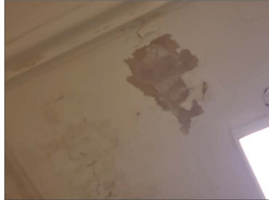
Water damage and cracks as seen below the interior of the roof at Bowie High School.
